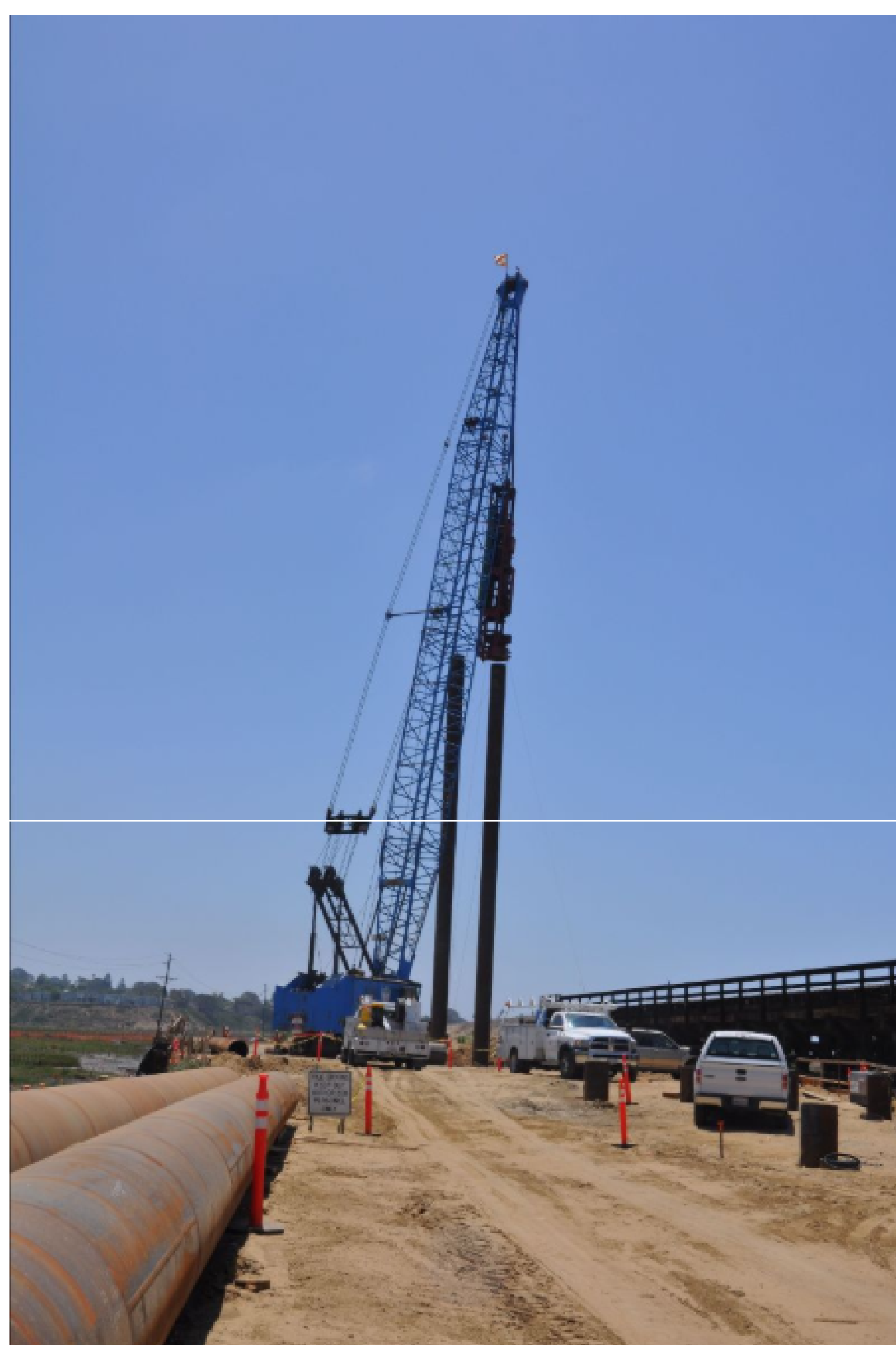
Example of active pile driving
